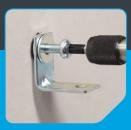
Tighten the screw until the fixing is secure.
