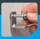
Insert the Stella-Fix screw through the fixing.
