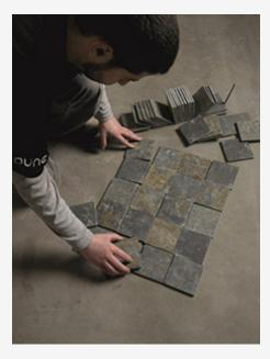
As we are dealing with natural materials, shade variation depends on the stone composition, which will be defined by the area of the quarry from which stone are extracted.
